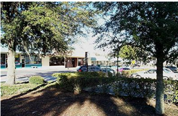
3_East_end_of_shopping_center_Small_ – East end of shopping center
